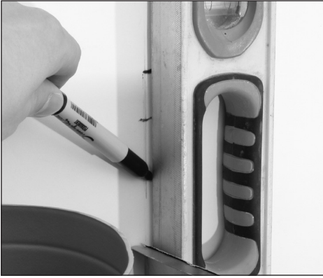
17. Mark out verticals along a straight edge, resting on the bottom half of the chimney
